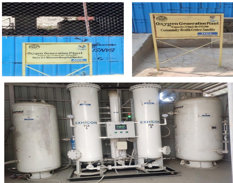
Figure 24: Oxygen plants set up in District Women's Hospital, Hardoi and CHC, Sandila
