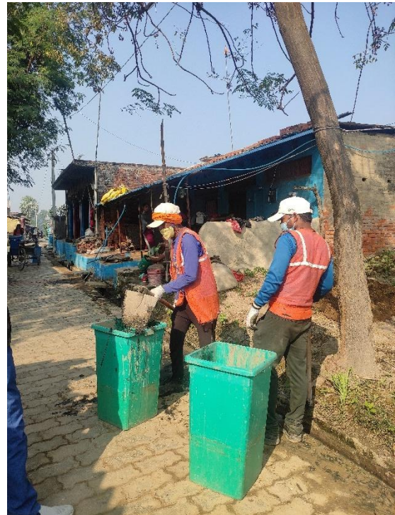
Image 6: Drain cleaning activity
